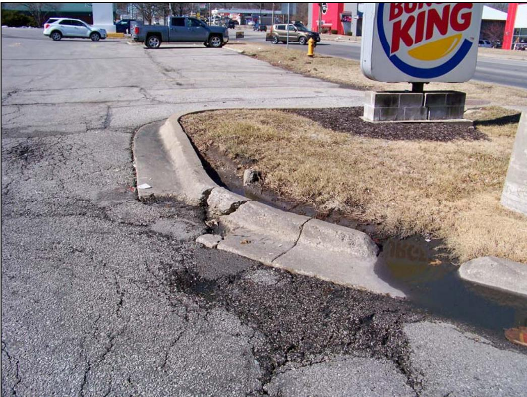
*Building 3 – looking west – deterioration of sign, curb, drive aisle; damaged landscaping*
