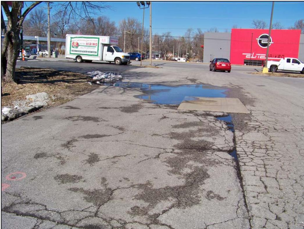
*Near Building 1 – looking north – deterioration of drive aisle; poor drainage*
