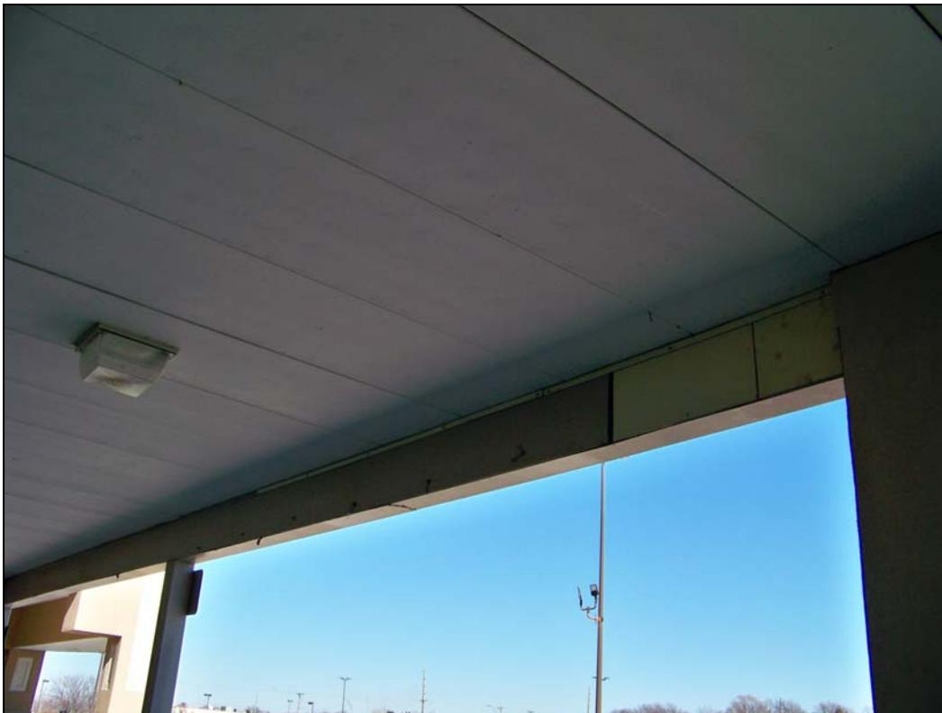
*Building 1 – looking northeast – deterioration of canopy beam and fascia*
