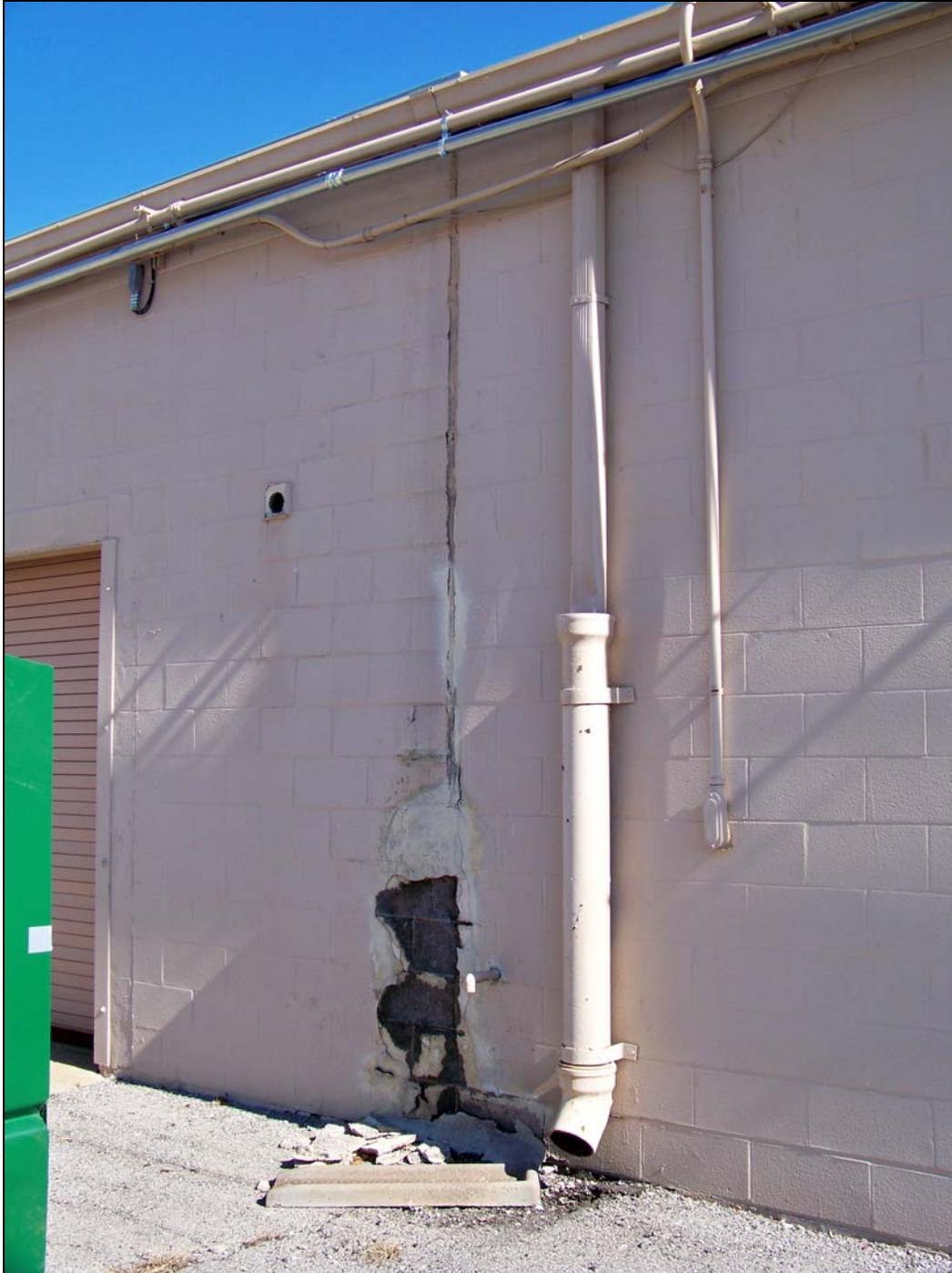
*Building 1 – looking east – deterioration of downspout, wall; failure of finishes*
