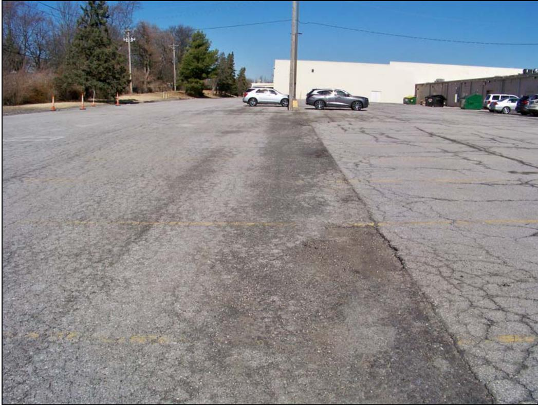
*Near Building 1 – looking north – deterioration of pavement*
