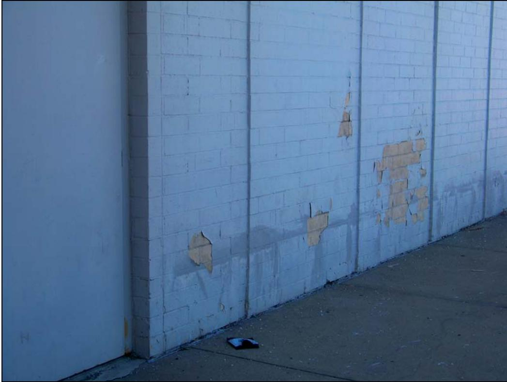
*Building 1 – looking west – failure of finishes*
