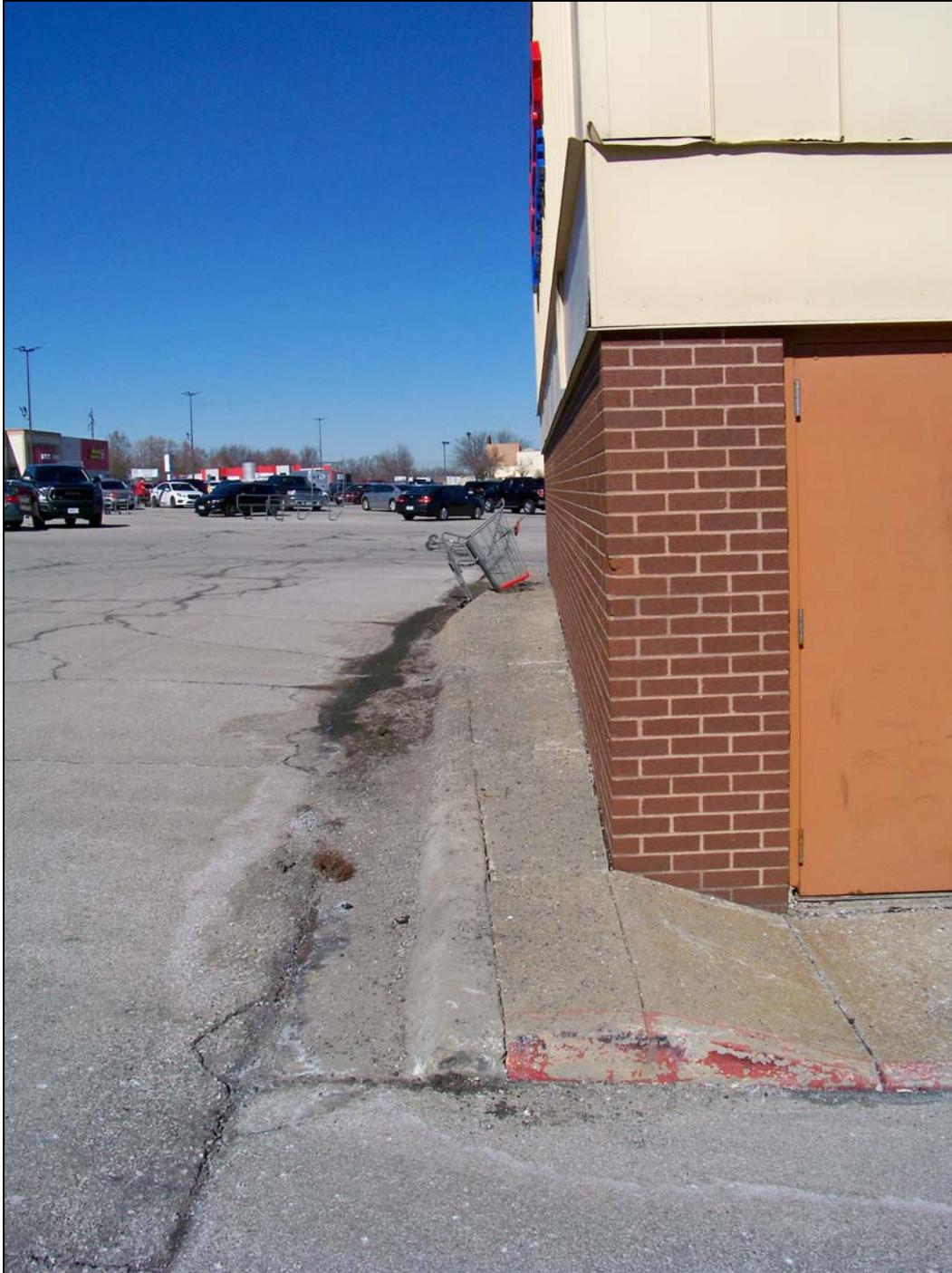
*Building 2 – looking north – deterioration of pavement and sidewalk*
