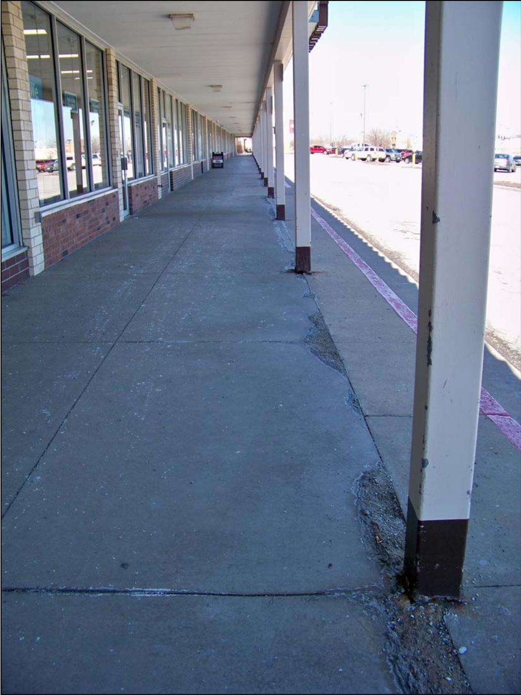
*Building 1 – looking north – deterioration of sidewalk*
