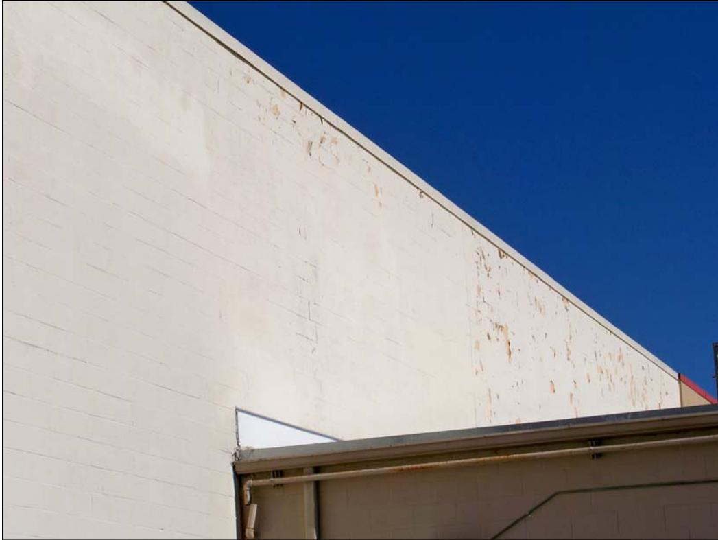
*Building 1 – looking north – failure of finishes*
