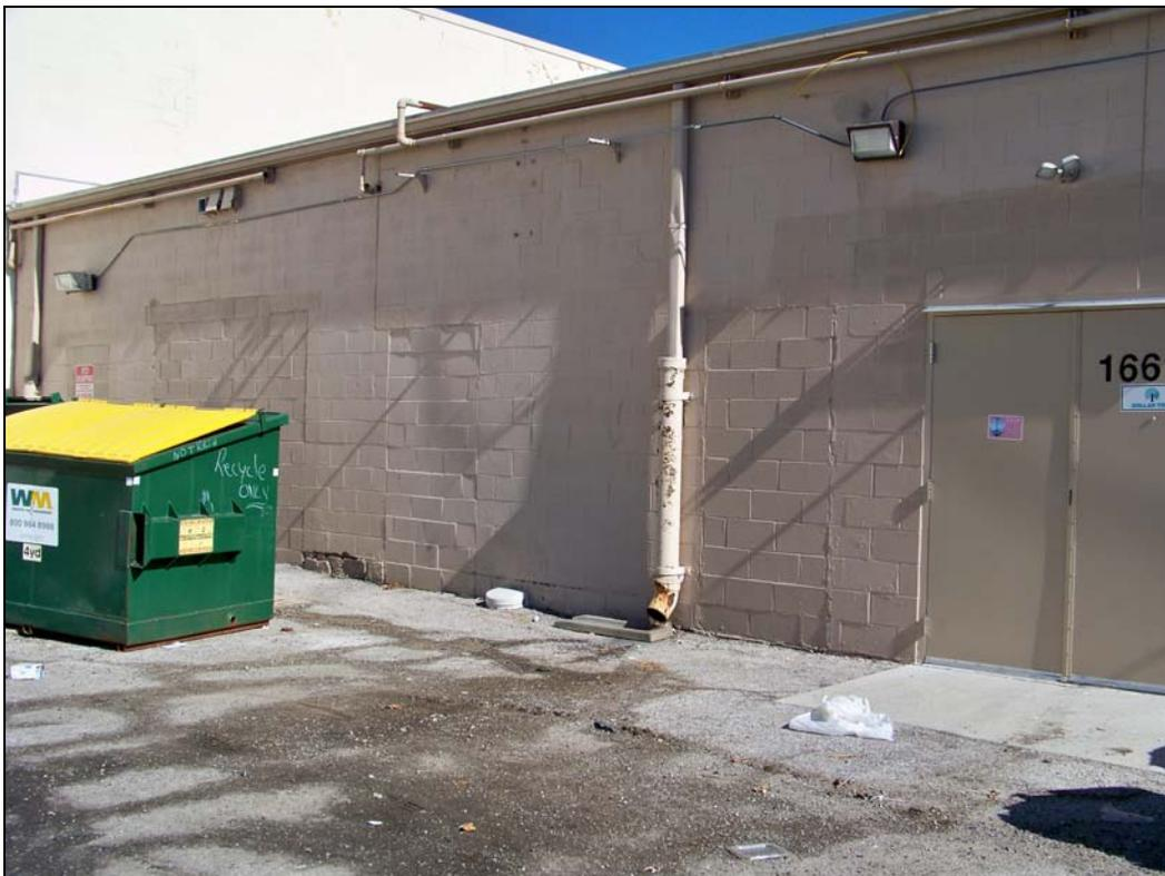
*Building 1 – looking east – deterioration of wall, gas line, downspout, pavement*
