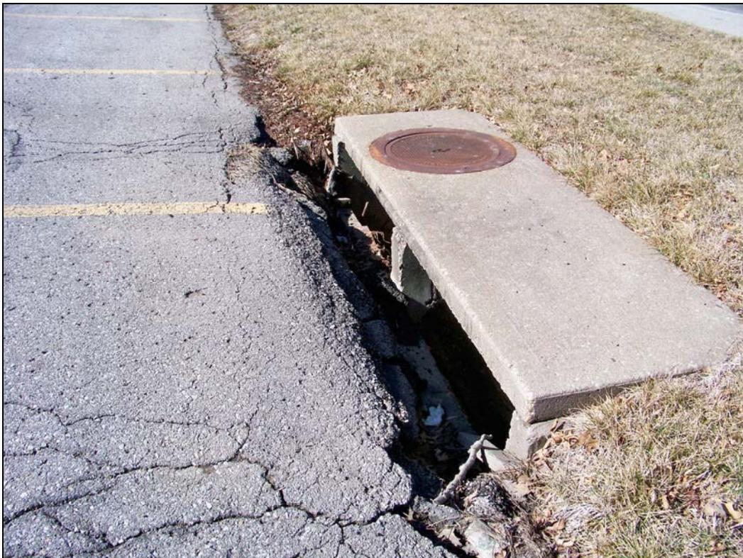
*Near Building 1 – deterioration of stormwater basin*
