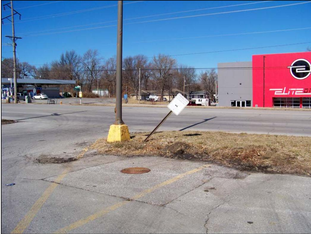
*Near Building 1 – looking northwest – deterioration of pavement, curb, signage; damaged landscaping*
