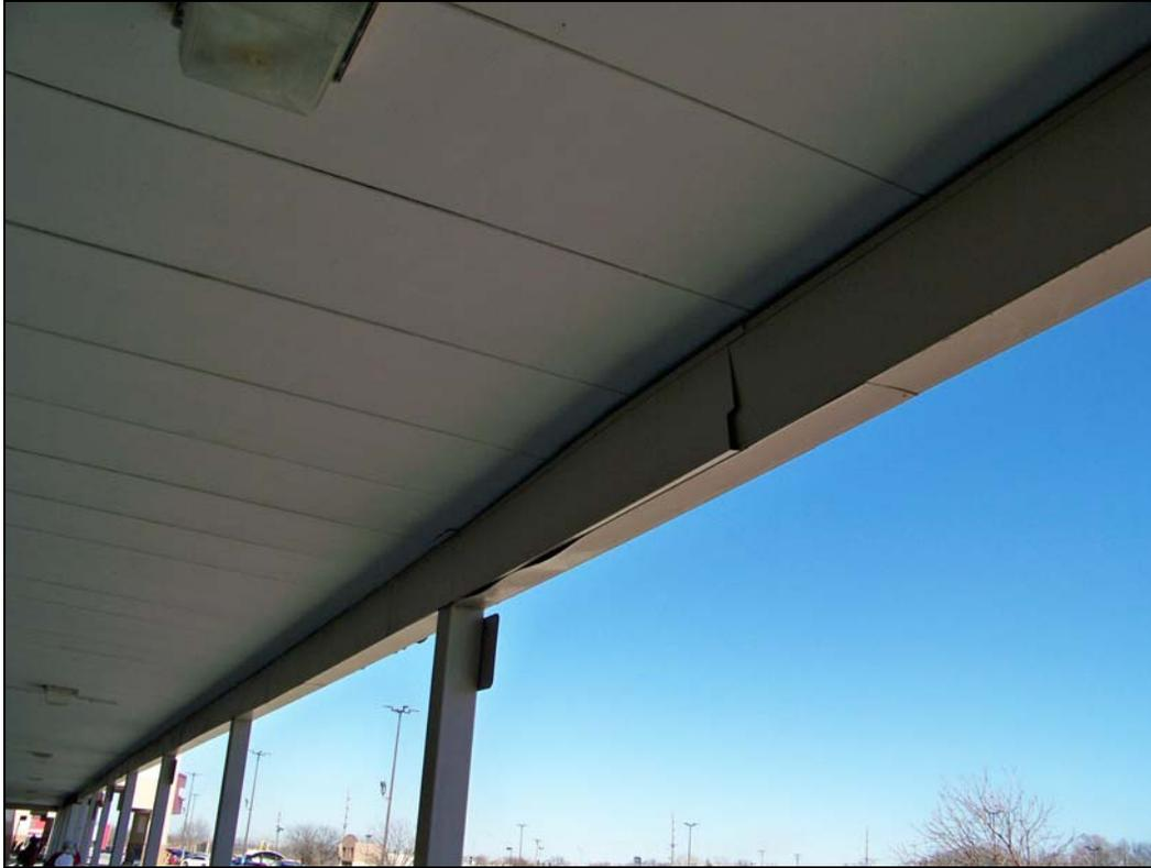
*Building 1 – looking north – deterioration of canopy beam and fascia*
