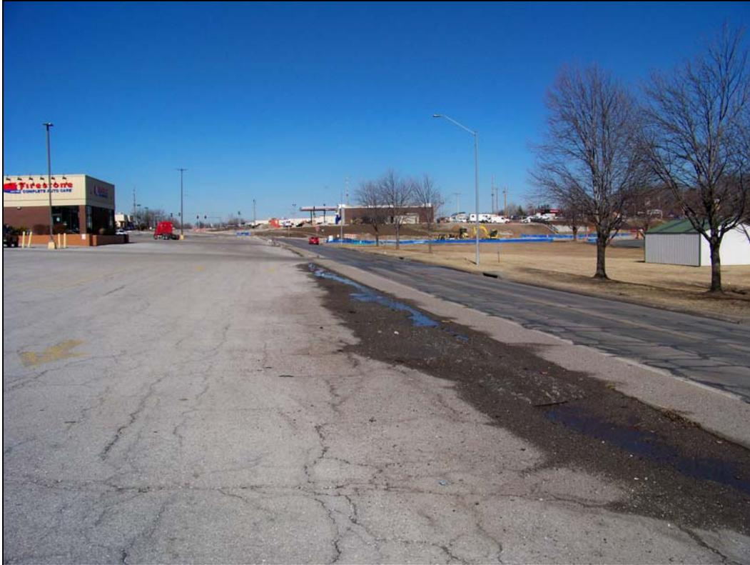
*Near Building 3 – looking north – deterioration of parking lot; poor drainage*
