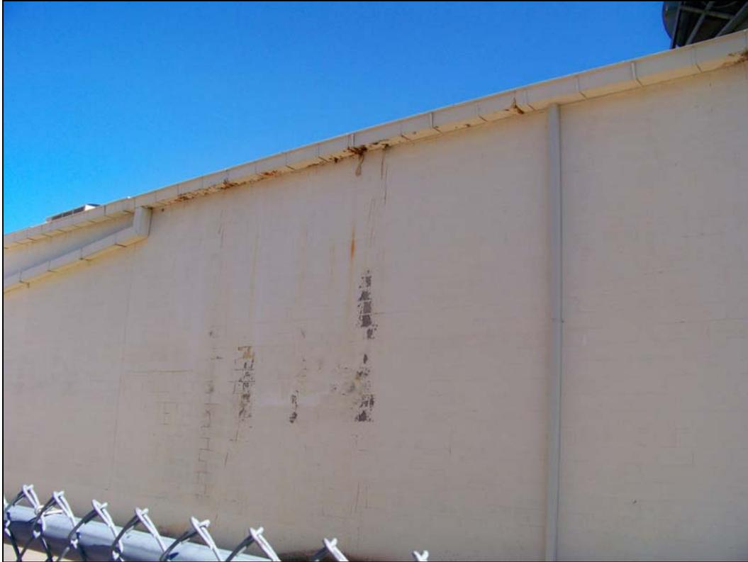
*Building 1 – looking east – deterioration of gutter; failure of finishes*
