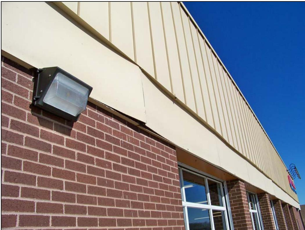
*Building 3 – looking northeast – deterioration of fascia, siding*
