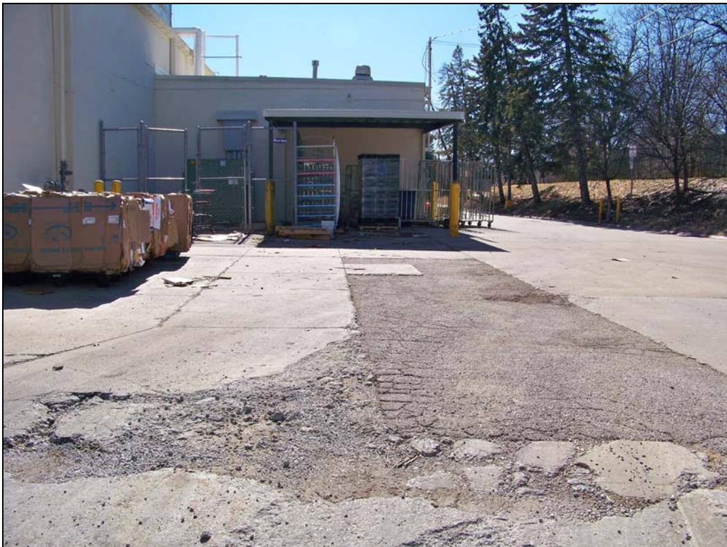
*Building 1 – looking south – deterioration of pavement*
