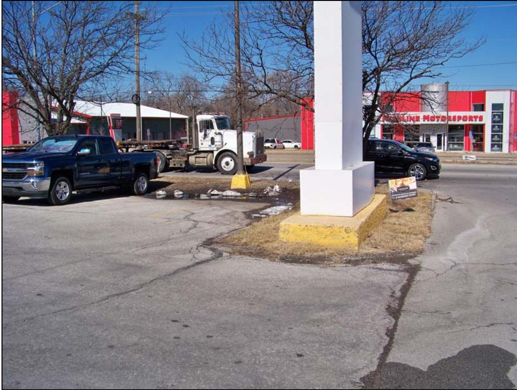
*Near Building 1 – deterioration of curb, parking lot; poor drainage*
