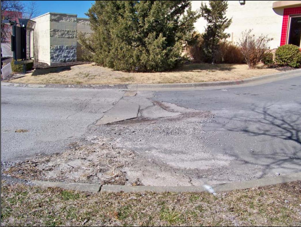
*Building 3 – looking northwest – deterioration of drive aisle*
