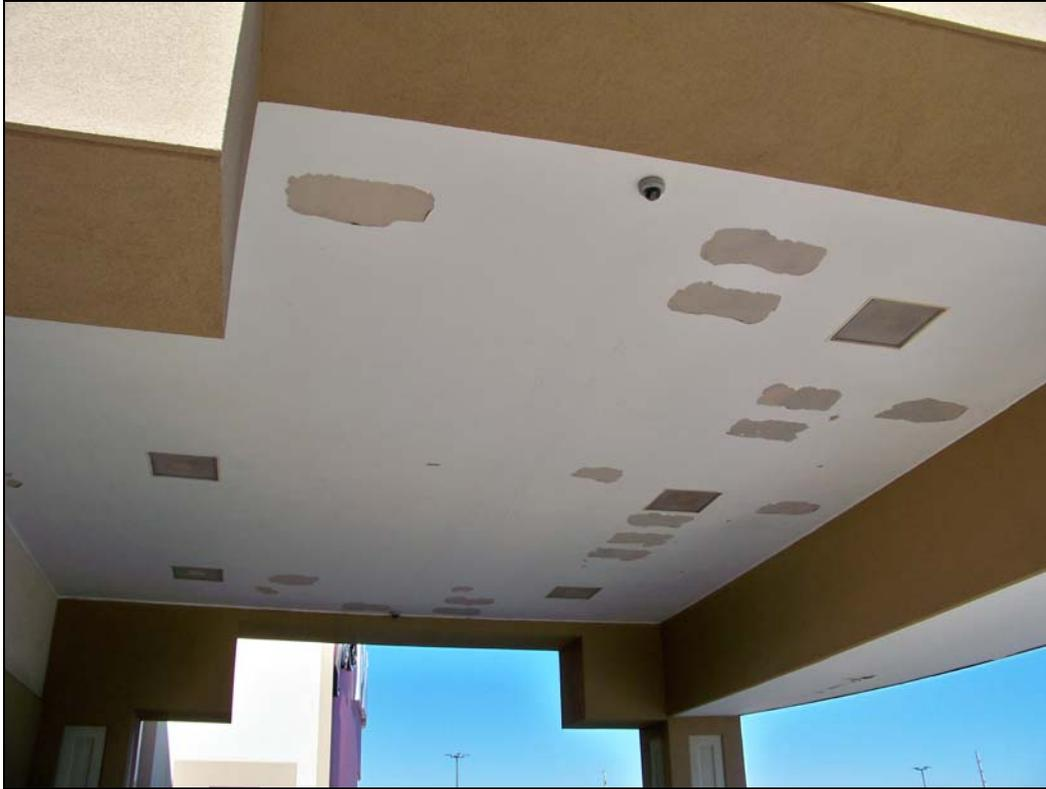
*Building 1 – looking north – deterioration of soffit; failure of finishes*
