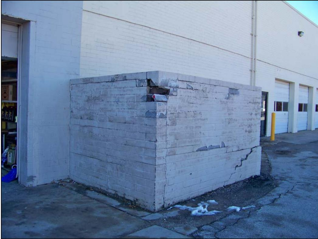
*Building 1 – looking southwest – deterioration of trash enclosure, parking lot pavement*
