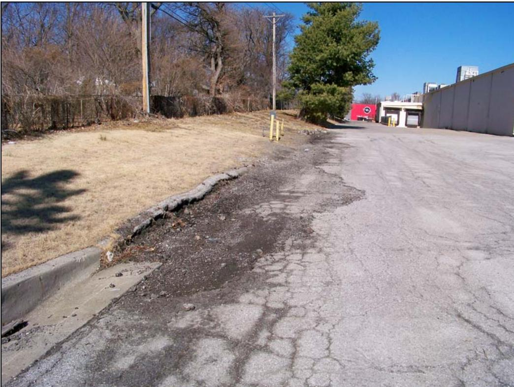
*Near Building 1 – looking north – deterioration of pavement, curb*
