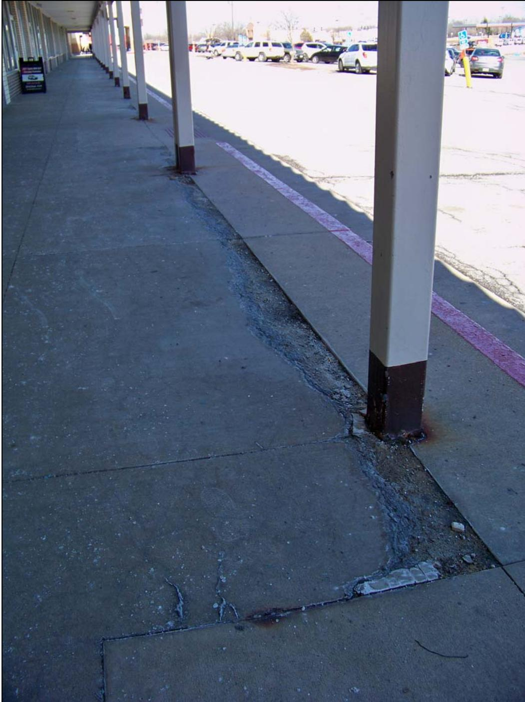
*Building 1 – looking north – deterioration of canopy columns, sidewalk*
