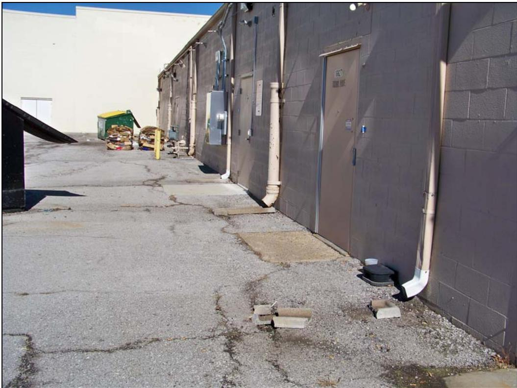
*Building 1 – deterioration of downspouts, pavement; failure of finishes; unenclosed dumpsters*
