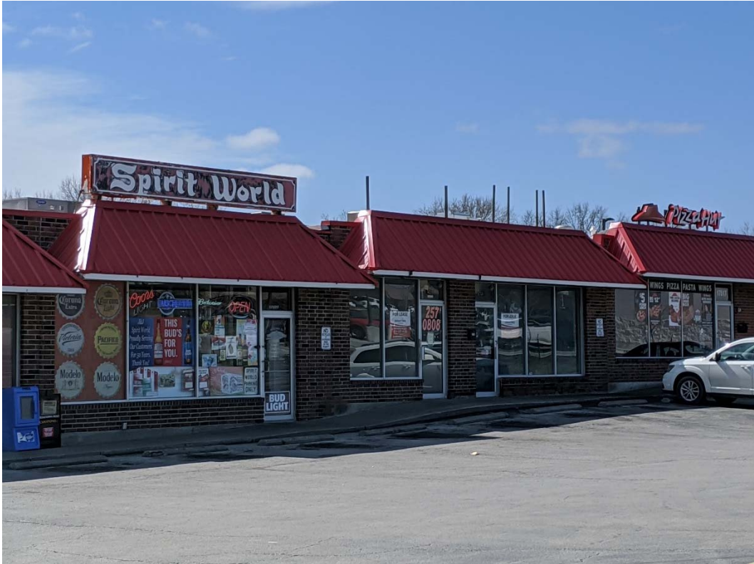
Legal nonconforming roof signs
