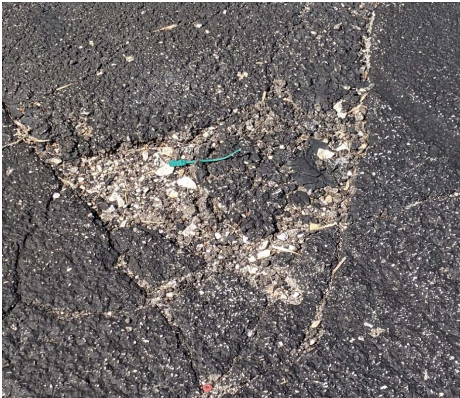
Deterioration of parking surface
