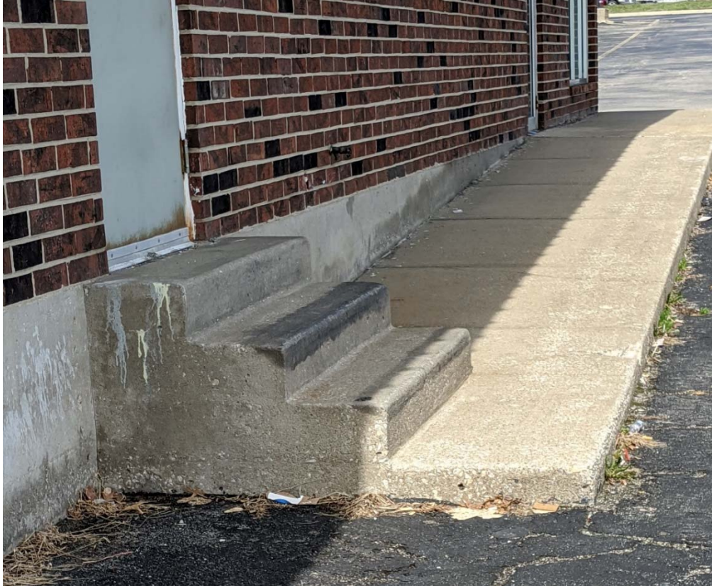
Deterioration of pavement and door
