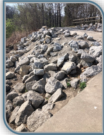
Washout repair with riprap installation at Waterfall Park
