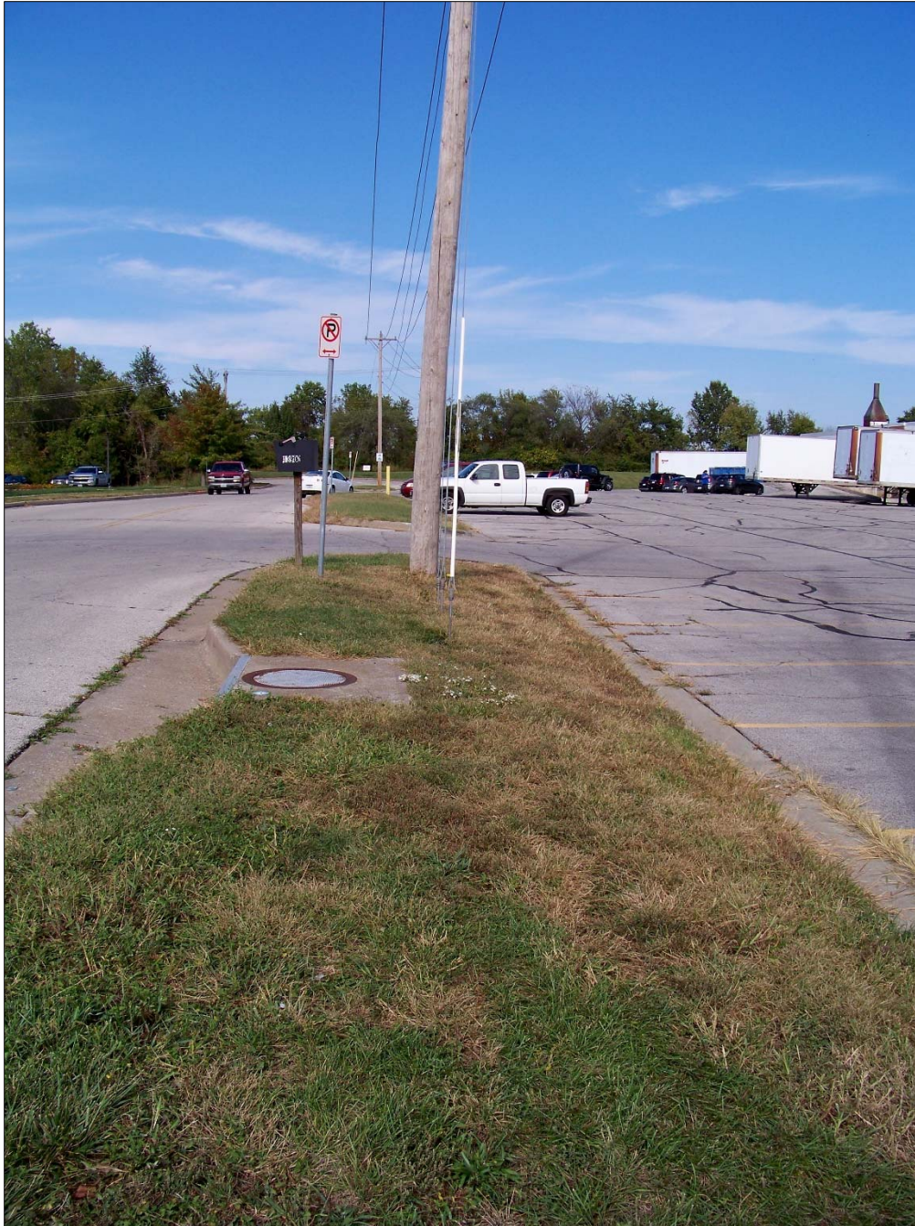
Lack of sidewalks
