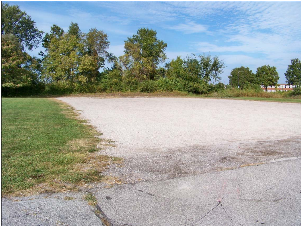
Gravel parking lot with no pavement markings, wheel stops, curbs at Cargo Largo building
