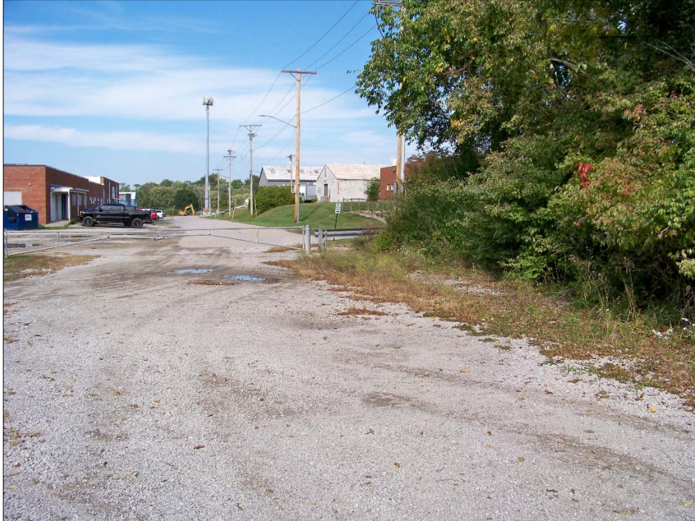
Deterioration of service drive at northwestern edge of Area
