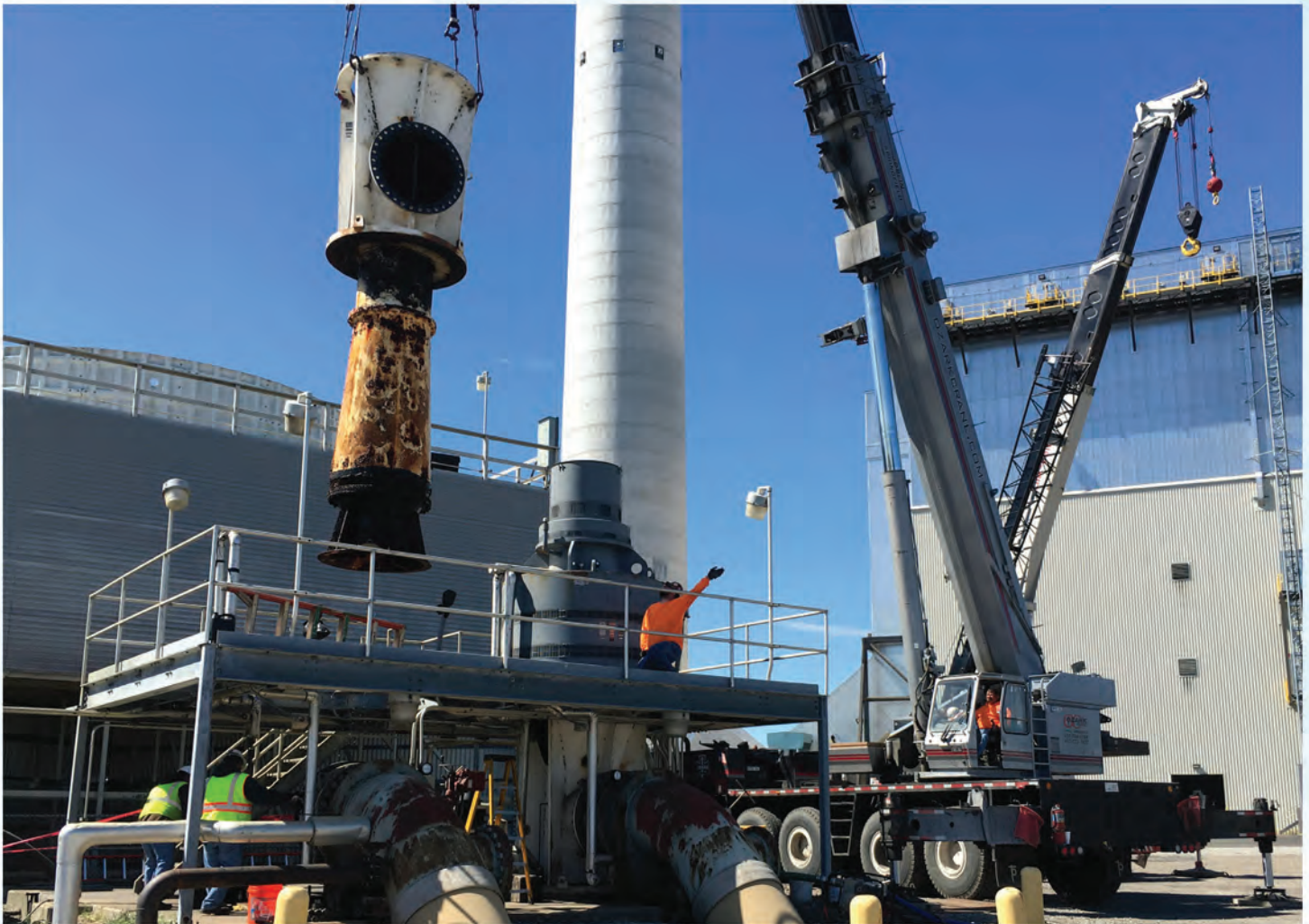
Field Service Removal of VTP
