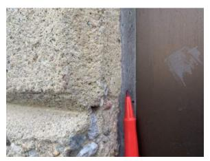
Image 10 – Deteriorated sealant joint.
