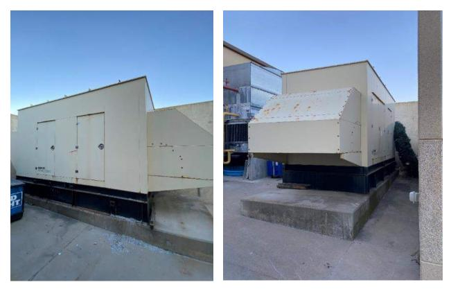
Image E-006 (left): Emergency Generator in service yard. Image E-007 (right): Emergency Generator air intake opening.
