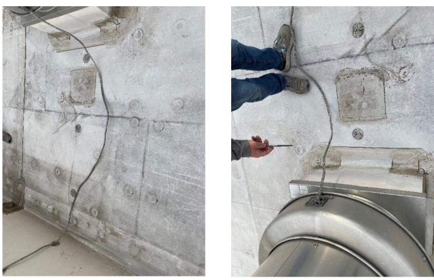
Image E-014 (left): Lightning Protection conductor free from Roof Cable Holder
