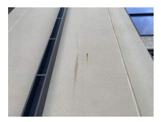
Image 14 – Hairline cracking in precast panel.
