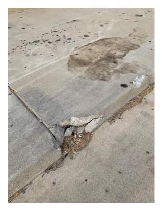
Image 4 – Spalling concrete at curb.
