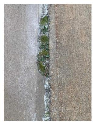
Image 5 – Spalling concrete at expansion joints.
