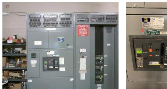
Image E-002 (left): MSB1-1 with single distribution section Image E-003 (right): MSB1-1 Main Circuit Breaker
