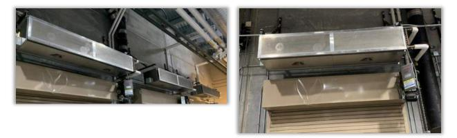
Natural gas fired, radiant heaters provide perimeter heating to the Community Ice Rink. Visual inspection of the heaters did not reveal any issues and appeared to be in good working condition. However, one of the heaters did have a flue pipe disconnected that needs to be repaired.
