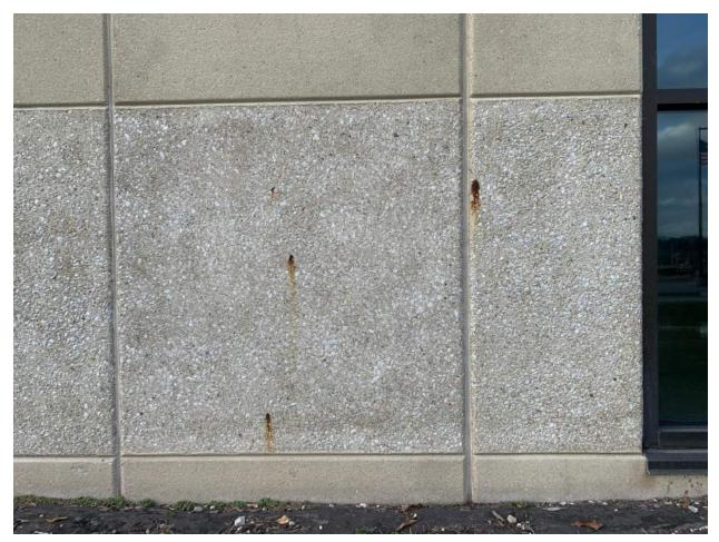
Image 15 – Precast concrete panels with rust staining.
