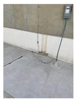
Image E-012 (left): Lightning Protection Air Terminal and Downlead Image E-013 (right): Lightning Protection Downlead and Thru-Roof Connection
