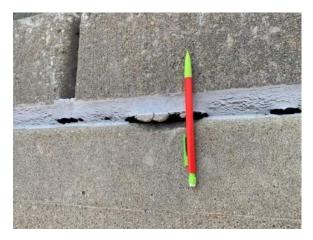
Image 3 - Failed sealant joint.
