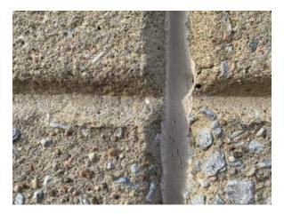
Image 16 - Deteriorated sealant at expansion joint.
