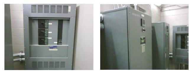
Image E-008 (left): Generator Distribution Board-GDP with (4) breakers for transfer switches Image E-009 (right): Automatic Transfer Switches: ATS-1 and ATS-2
