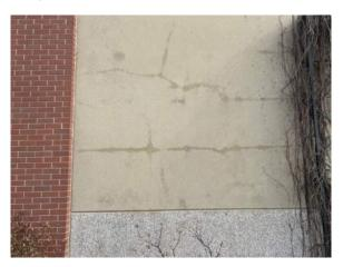
Image 19 – Hairline cracking in stucco.
