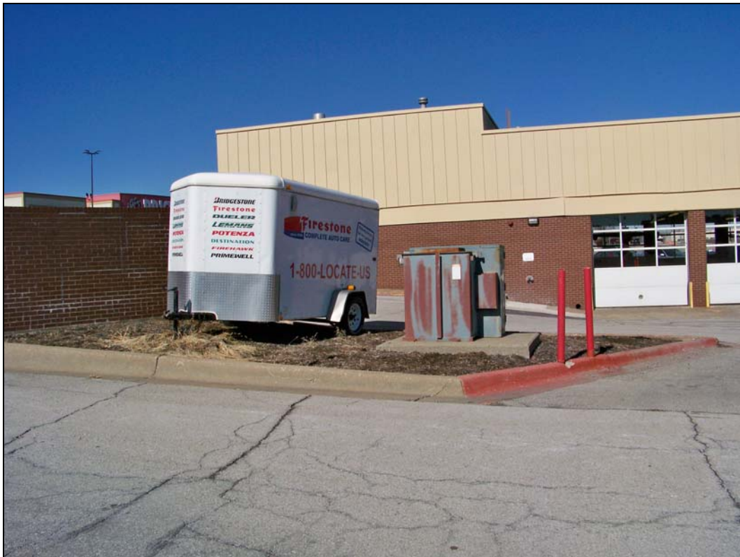
Building 3 – looking north – deterioration of equipment
