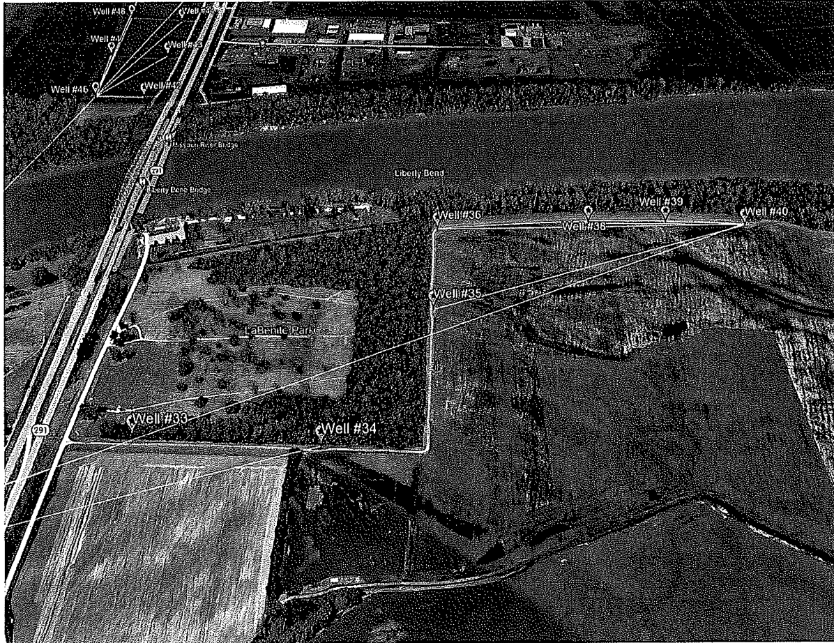
Picture 3 –East Wellfield area radio network
